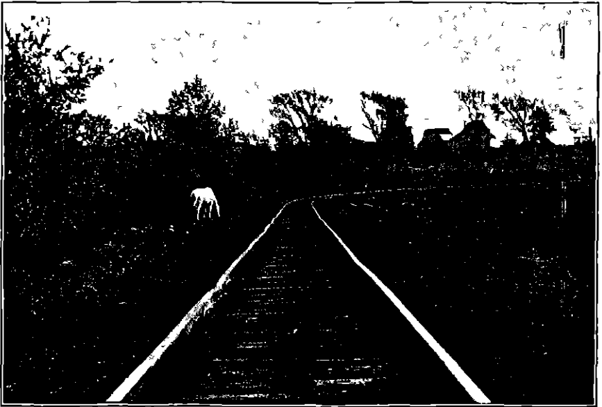
No 2—View of track south of point of accident
