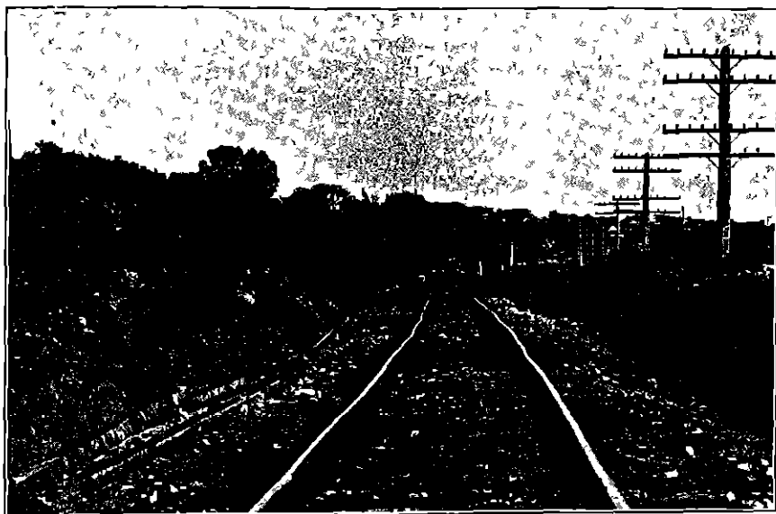
No 1—View of track approaching point of derailment from the north
